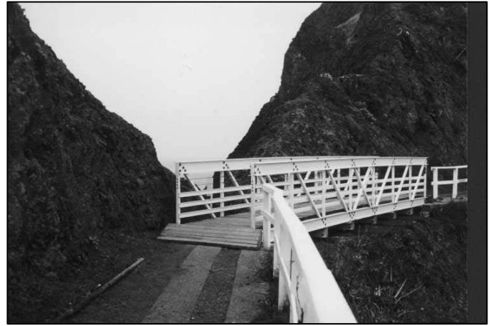
Bridges are easily installed in hard-to-access areas.
